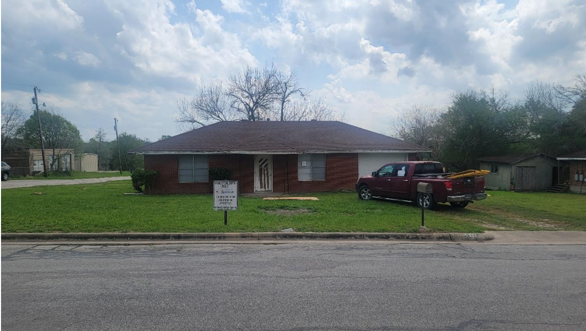
803 Matchett Street- Existing home being remodeled.
